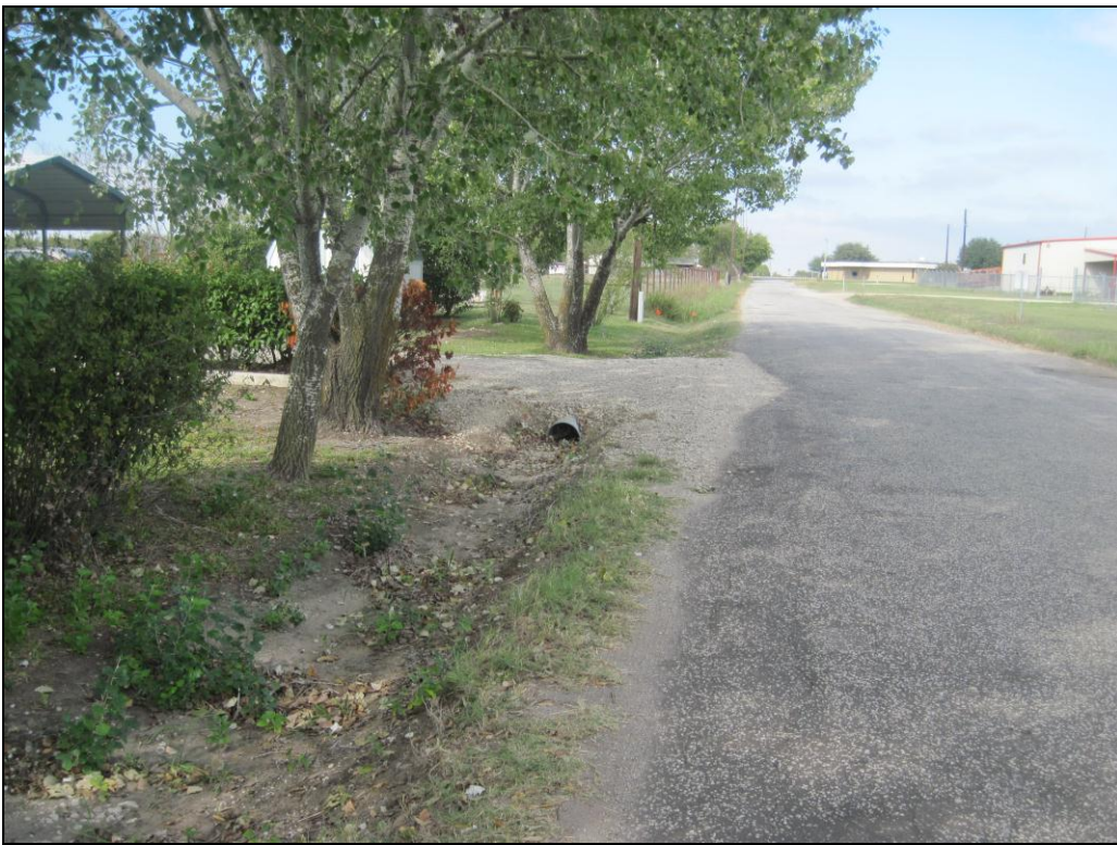
Figure 7B: Shallow drainage channel
