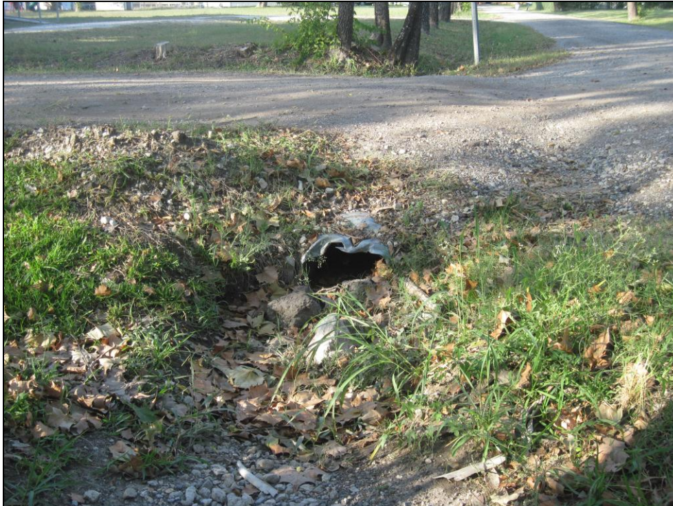
Figure 7D: Damaged CMP (Elm St. and Windsor St.)
